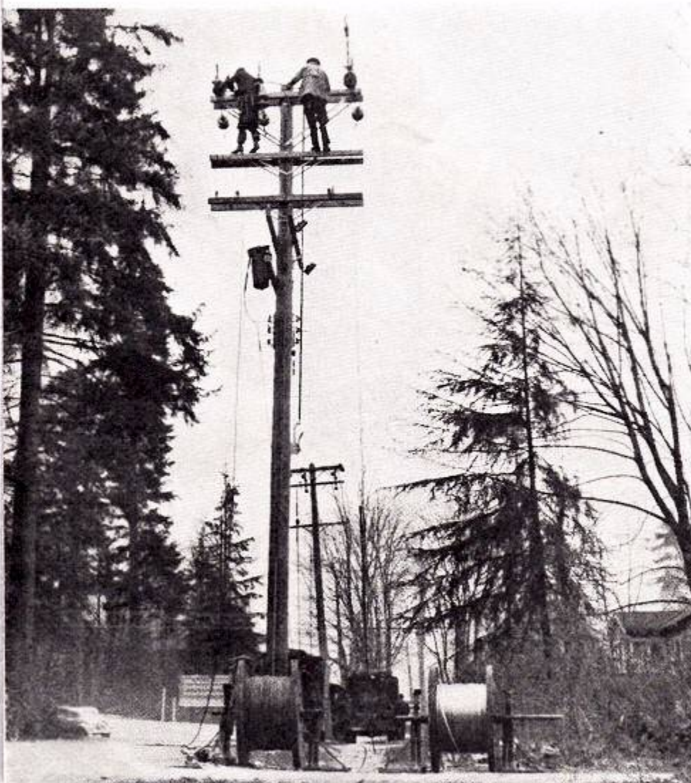
A COUPLE of Bill McLennan's linemen during recent construction on the new 12,000 k.v. line at Keith road and St. Denis.
