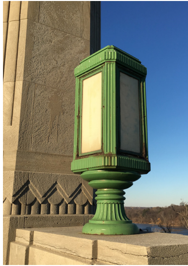
High Level Bridge lantern
