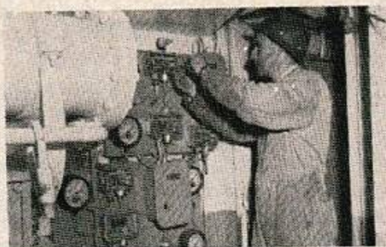
Shop 05, Refrigeration Shop — Roy Bannister , refrigeration mechanic adjusting the controls of the main refrigeration machinery on board ship.
