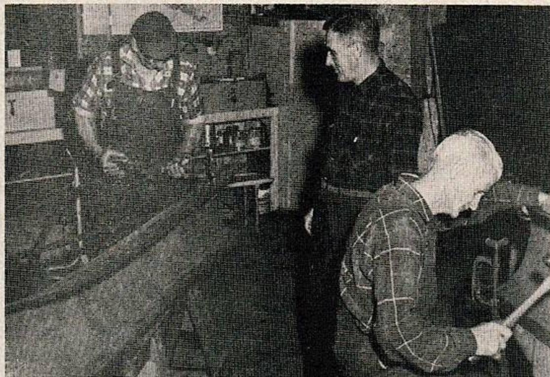
Shop 04, Pipe Shop —Art Storey supervising the fabrication of a 14" diameter pipe from 14 gauge copper. This pipe is made by hand in two sections which
