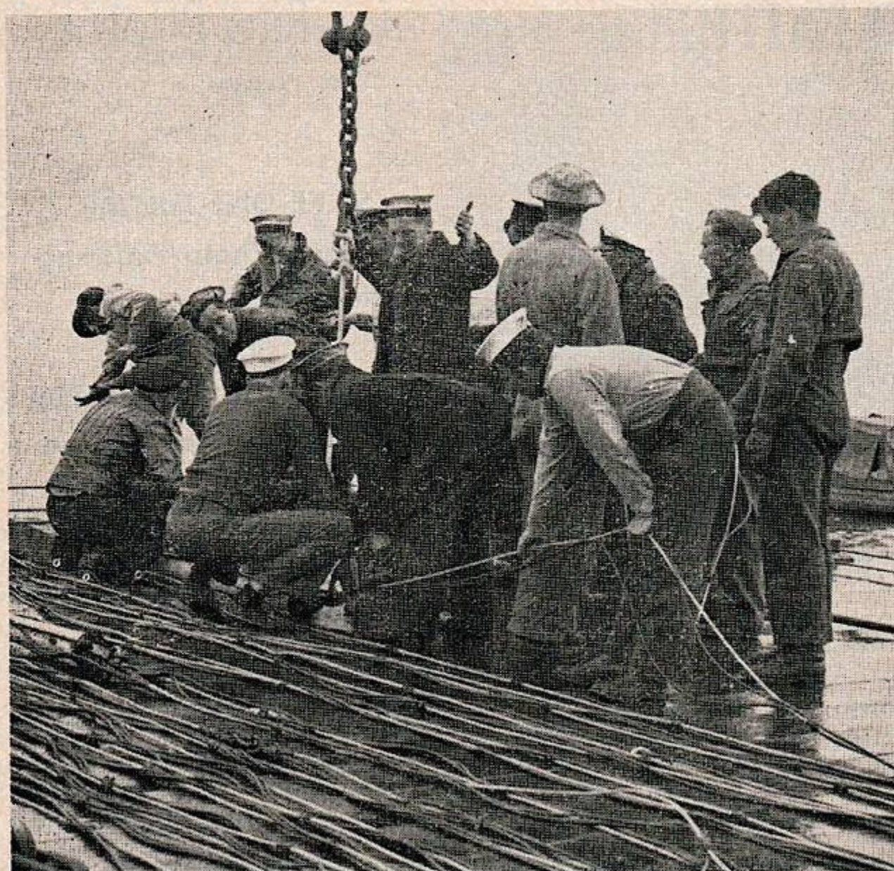
Lowering a set of underwater listening coils off Whitecliff, Howe Sound, for NRC. RCN Photo E6168
