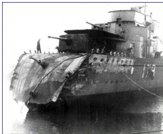
Torpedo damage December 1940
