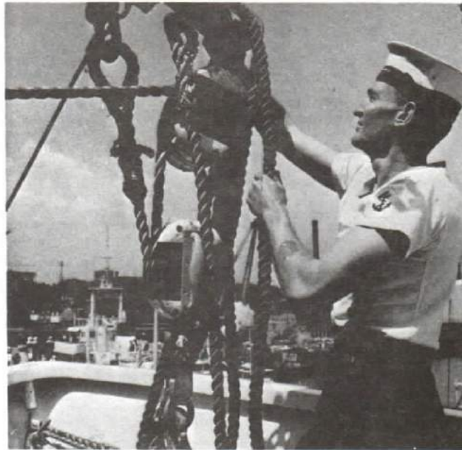
Figure 12-27 Passing Second Bight Passage du second tour
