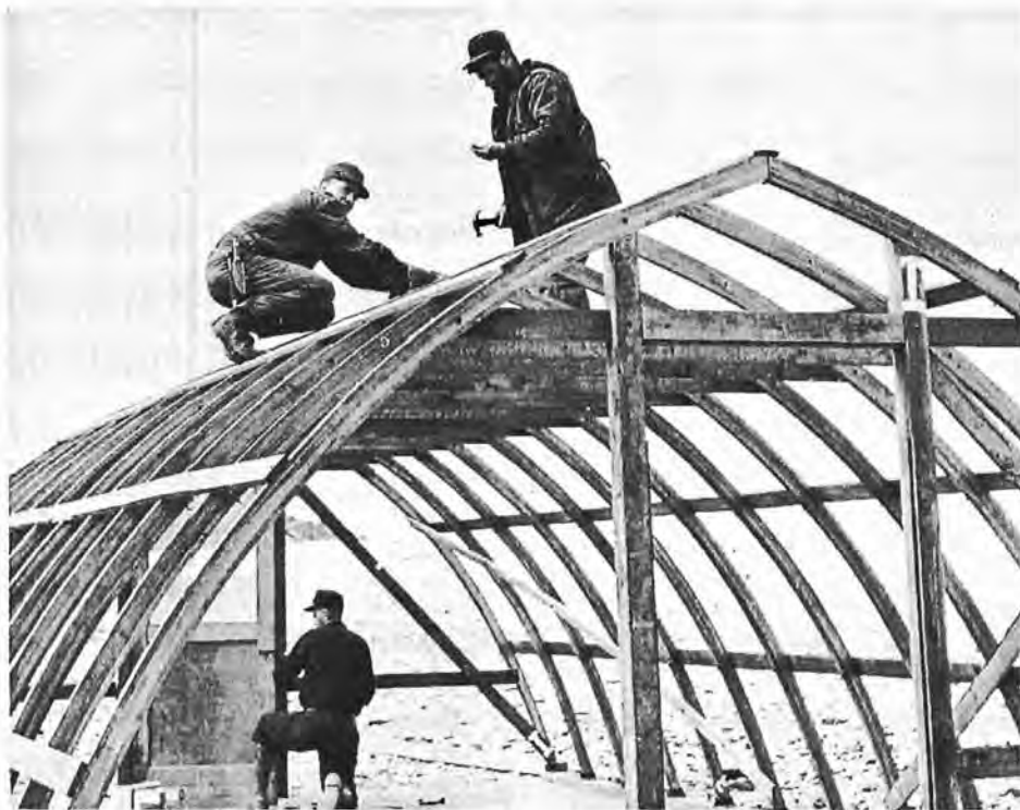
Flown from the Labrador by helicopter over miles of ice-clogged sea, an Atwell shelter to house personnel operating electronic position indicator equipment is assembled by Able Seaman Burton Reid and Walton Chipman and (below) CPO Riley Mombourquette. (LAB -930)
