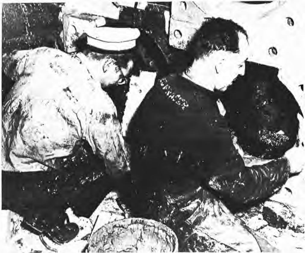
Happy although the lot of the man in the boiler room may be today compared with his existence in the coal-burning era, there are still a few important jobs which are a bit on the messy side. This picture is of brickwork being repaired in HMCS "Huron's" No. 3 boiler during her first tour of duty in the Far East. (HU-75)
