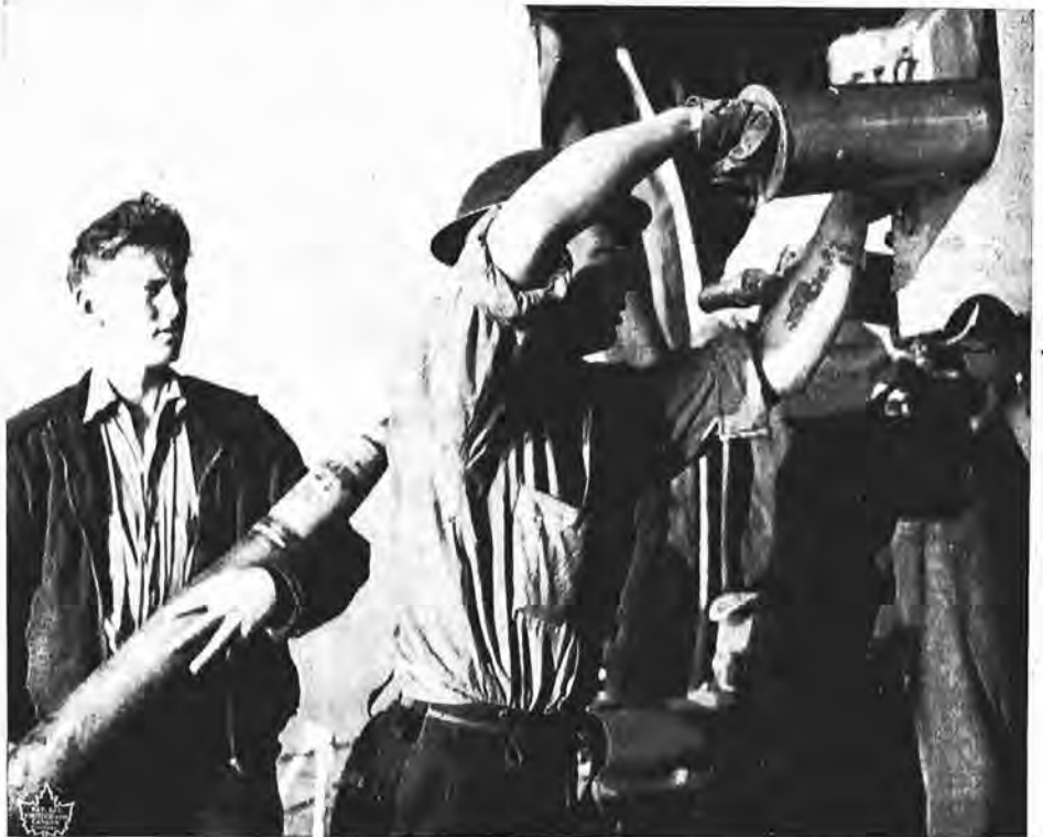
In this photo, AB Beech loads round number 7,322 while AB Robertson stands by with number 7,323 — the last shell to be fired by the "Athabec". (AN-94. All photos by Ldg. Sea. G. J. Brown).
