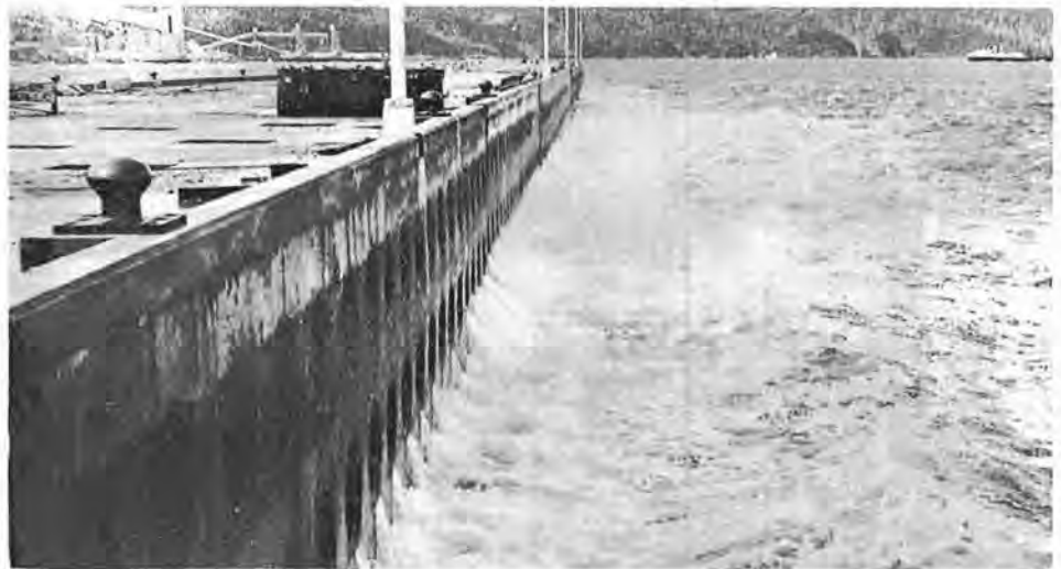
A perforated caisson breakwater-wharf—the world's first—is in operation at Baie Comeau, Quebec. The breakwater is honeycombed with holes through which large waves pour into a chamber where their energy is dissipated by friction and turbulence, and the force of succeeding waves is broken by outrushing water. The top picture is an offshore view of the wharf. In the middle picture a caisson is being towed into position. The bottom picture shows water from spent waves pouring back into the St. Lawrence River, which is about 35 miles wide at that point. (Department of Public Works photos)
