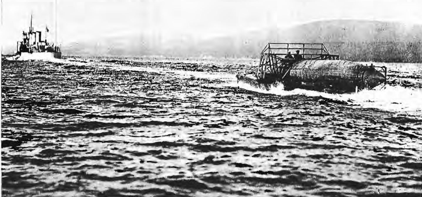
The Royal Canadian Navy's interest in hydrofoil development goes back to the years just after the First World War. HMCS Patriot, a destroyer, is shown towing at 14 knots the HD-4, a hydrofoil craft designed by Dr. Alexander Graham Bell and F. W. (Casey) Baldwin, on the Bras d'Or Lakes, near Baddeck, N.S. The HD-4 established a 60-knot speed record that stood for a generation. (CN-2947)
