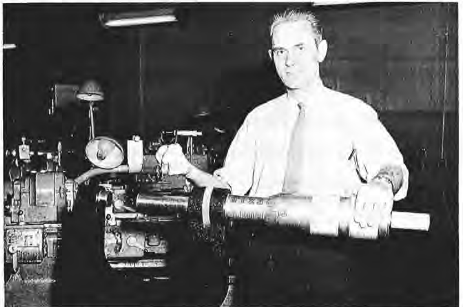
G. K. Lloyd, instructor in the Machine Shop of the Academic Division of the Fleet School at Stadacona, produced this 1-10 scale micrometer to enable trainees to grasp more readily the fundamentals of the device. It can be readily seen from the rear of a classroom and has proved an invaluable training aid. (HS-61893)
