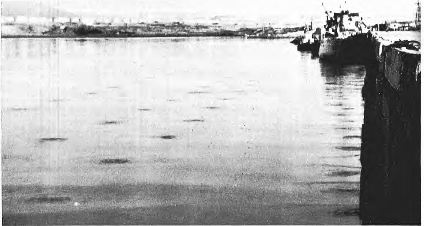
The pattern of disturbed patches on the smooth surface of Thule Harbour, in Greenland, indicates that the polynia system, installed with the assistance of RCN divers, is functioning as it should. The slightly warmer water of the harbour bottom is carried to the surface by air bubbles to prevent the formation of ice. (Official U.S. Navy Photograph)
